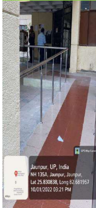
Ramp at the Administrative building
